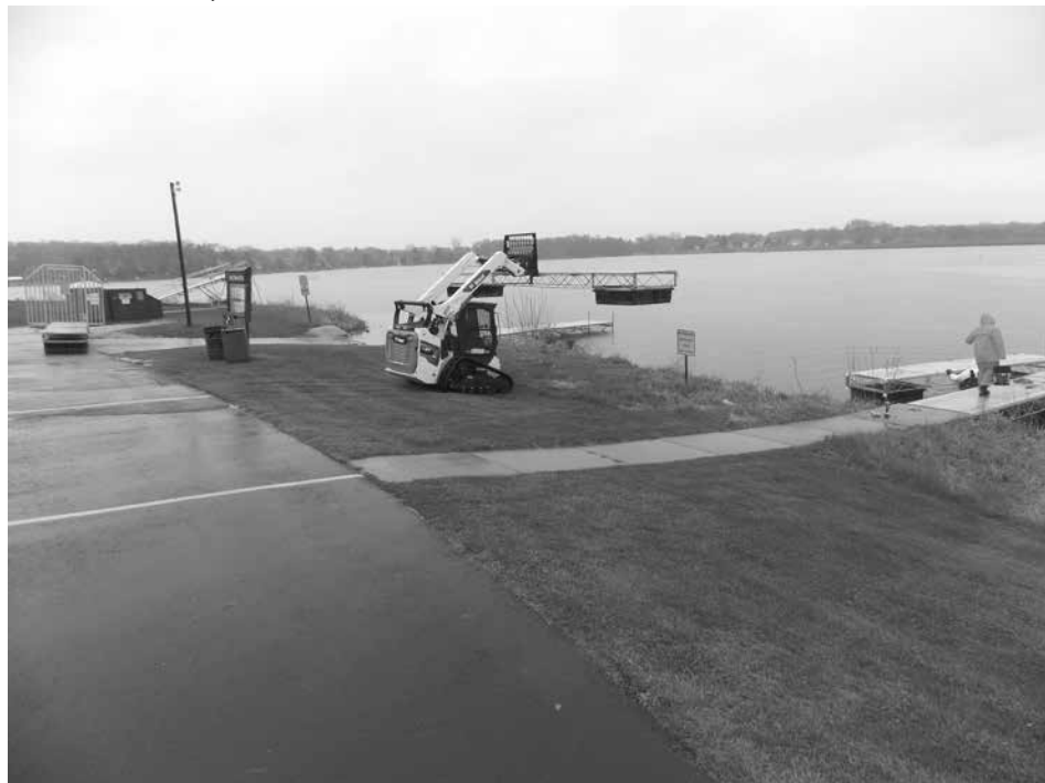
Bobcat bringing pier sections to the water.
