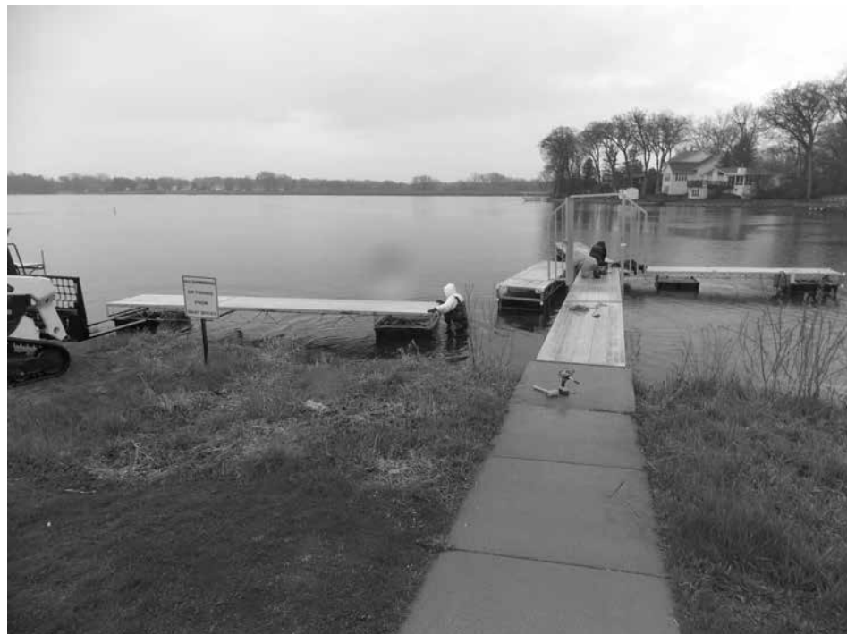
Two men in the water assembling dock A.
