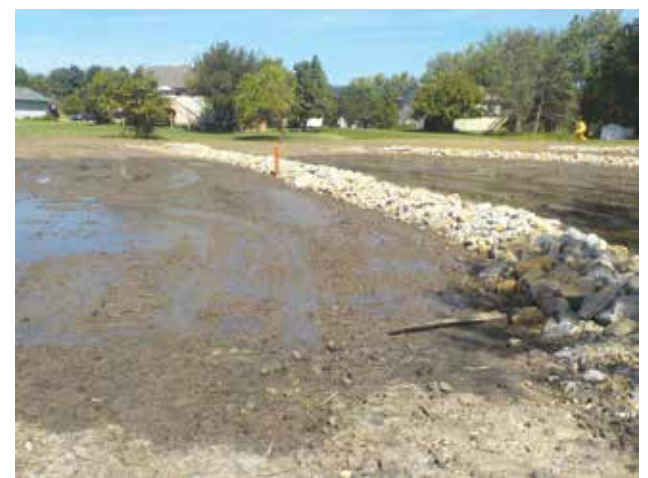
All these step down pools will be seeded with nutrient hungry plants, much like our swales.
